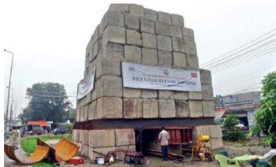
Fig.4 Concrete Blocks Platform at Orange Line Metro Train Project, Lahore
